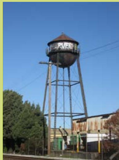
Water tower near 49 th Ave
