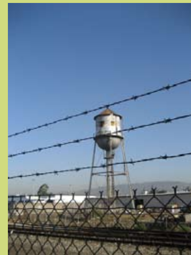
Water tower near 60 th Ave
