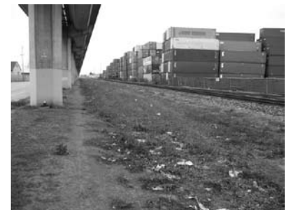
A simulation of a vegetated swale in Oakland under the BART columns using upper easements
