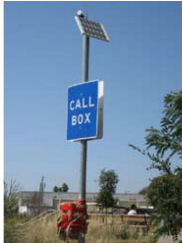
Solar powered call box on the Ohlone Greenway
