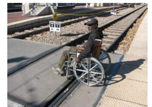
Pedestrian railroad crossings need to be accessible, with a reubberized surface or concrete slab insert.
