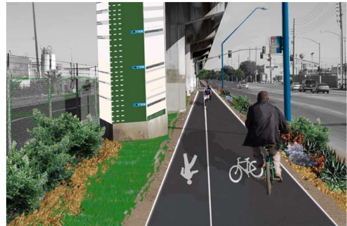
Rubberized asphalt, a Class I bikeway, BART column signage, and 2-foot wide soft shoulders are shown in this simulation of the Greenway at 81 st Avenue in Oakland
