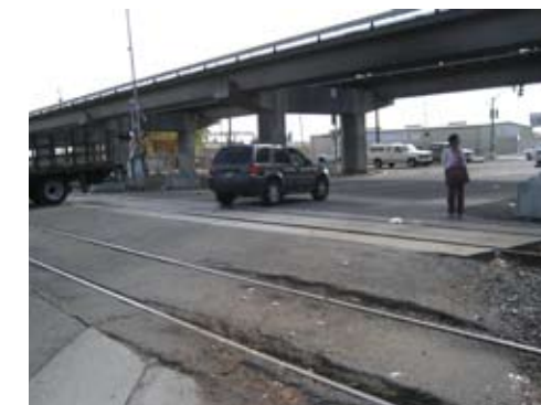
Existing railroad track crossing in Oakland
