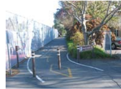
Removable bollards with striping and reflective markers stops vehicles from driving on the Greenway.
