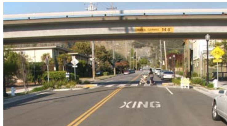
Midblock crossing on the Ohlone Greenway
