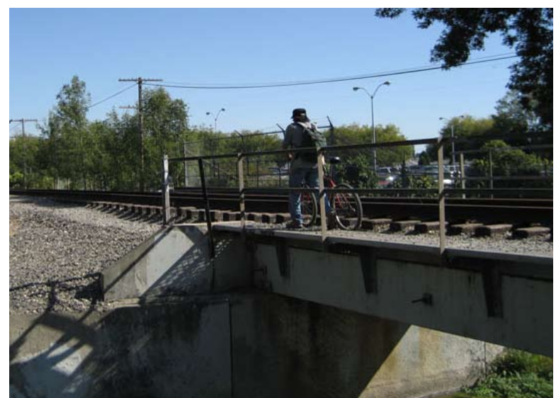
Bike crossing Estudillo Canal near Bay Fair Station
