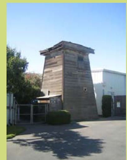
Tankhouse near 143 rd Avenue
