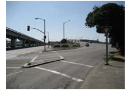
22 nd Avenue intersection
