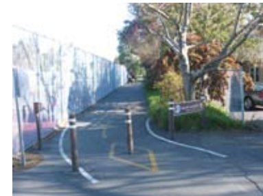
Removable bollards with striping and reflective markers stops vehicles from driving on the Greenway.
