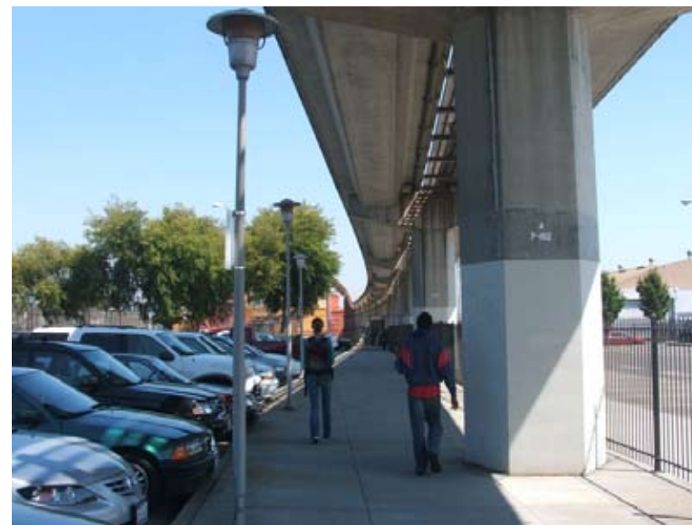
Sidewalk underneath BART tracks in BART parking lot
