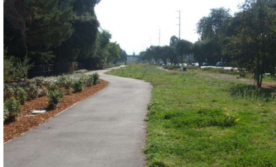
Iron Horse Trail, between the cities of Concord and Dublin, follows the old Southern Pacific Railroad right-of-way
