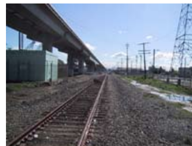
BART switching station near Washington Avenue
