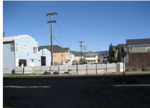
Access to the Greenway blocked by UPRR land
