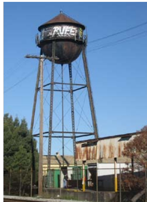
One of the many water towers that dot the East Bay Greenway route
