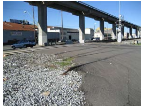
Existing condition of the railroad crossings
