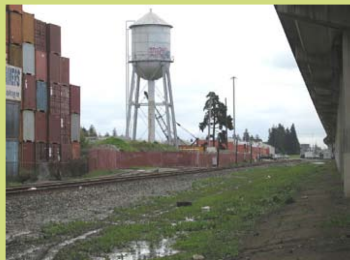
Water tower near 98th Avenue
