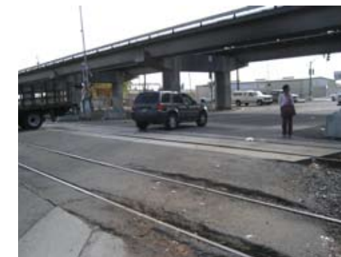
Existing railroad track crossing in Oakland
