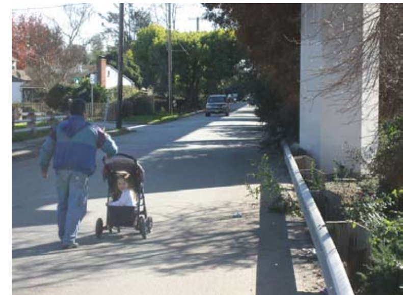
No sidewalks are available on the east side of Western Boulevard
